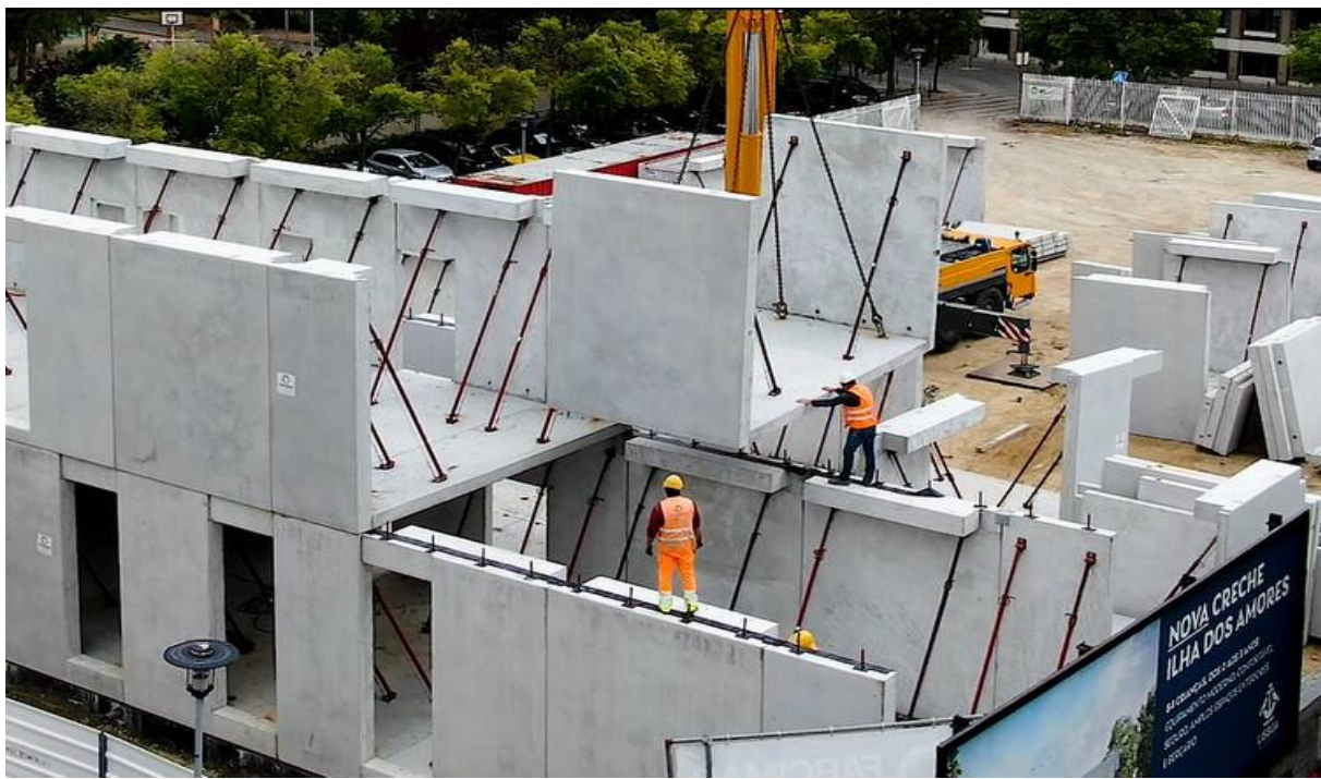
Figure 2-6:Installation of precast elements in a housing project
