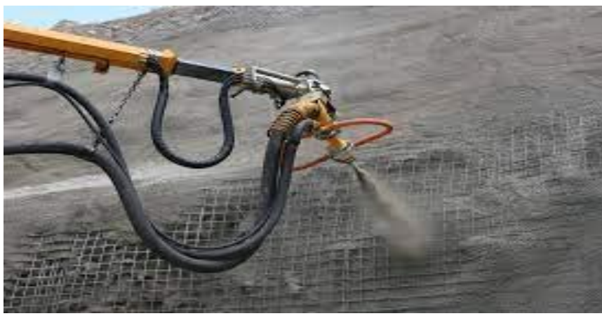
Figure 2-8: The process of pouring shotcrete for a concrete wall
